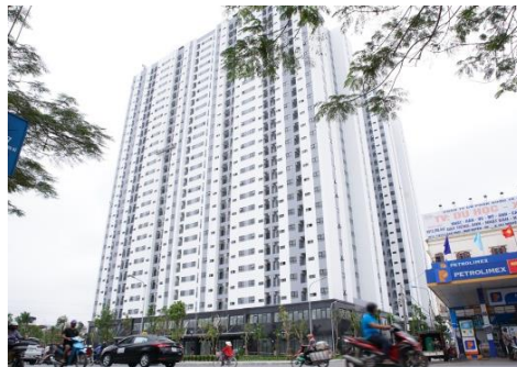
Apartment complex HH3, HH4
